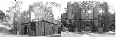
Water conservation is emphasised by building this house using recycled plastic bottles that conserves water, as opposed to traditional building materials like concrete that require more water usage. ☑ The use of these water bottles to build ensures that they do not find their way into our oceans, rivers and dams. ☑ The use of recycled plastic in FIGURE L enhances the importance of water conservation by highlighting the use of recycled water bottles. ☑
